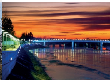
8 Bridge over the Tanaro
